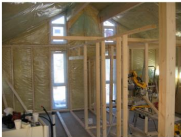
Building structure finished, Inside work on track
