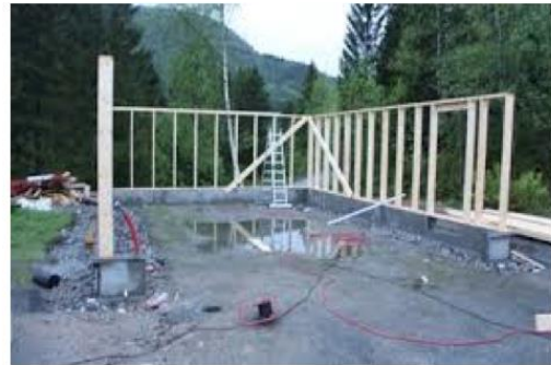
Foundation finished, building structure started
