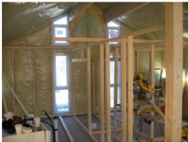
Building structure finished, Inside work on track
