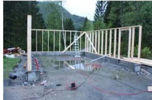
Foundation finished, building structure started
